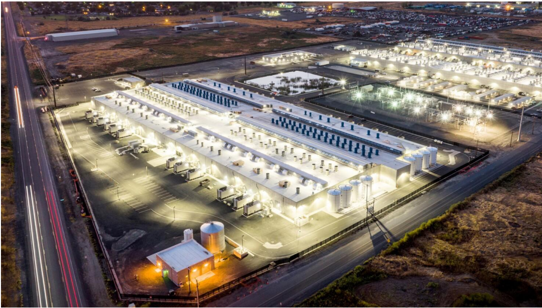
292 Figure 2. Image of the Amazon data center in Oregon, United States
